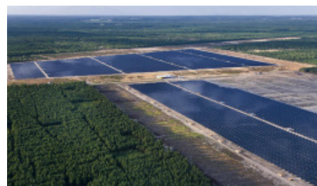
Figure 8: Lieberose PV park, Germany, © www.solarserver.de
