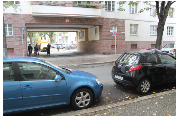
(d) T-shaped intersection with missing crossings via through street (Ilsestraße/Ilsenhof)
