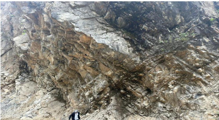
Photograph 5: Rock fall chances in the mining sites near Roshi Khola.
