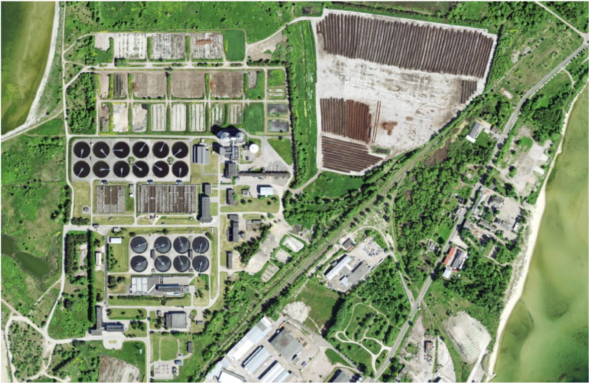
Figure 22: Large industrial area in Tallinn.
