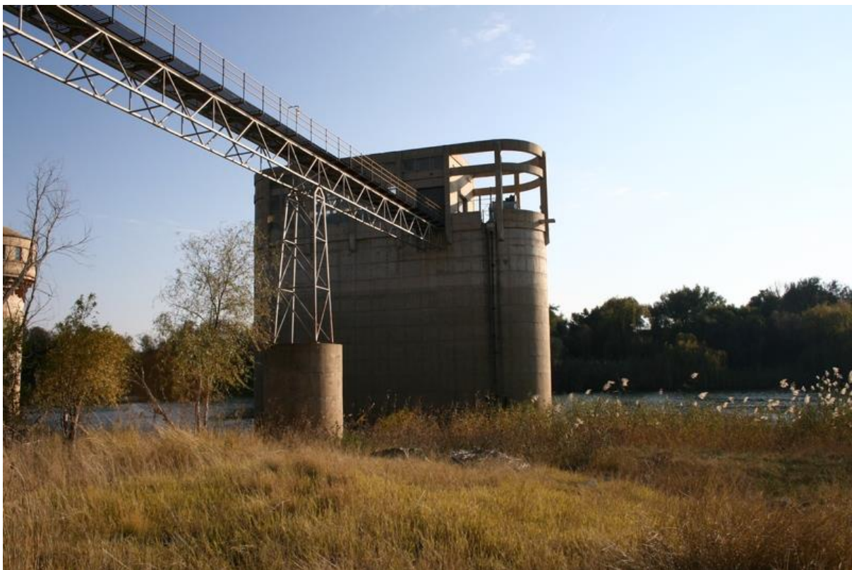
Figure 3-4 Riverton waterworks station(Department of Water Affairs n.d.).
