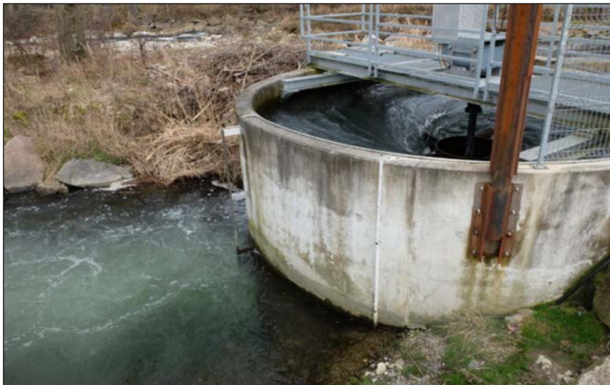
Figure 1-3: Vortex energy plant "Dr. Bertrand Piccard", Schöffland AG, Switzerland (Source: Verde Renewables).
