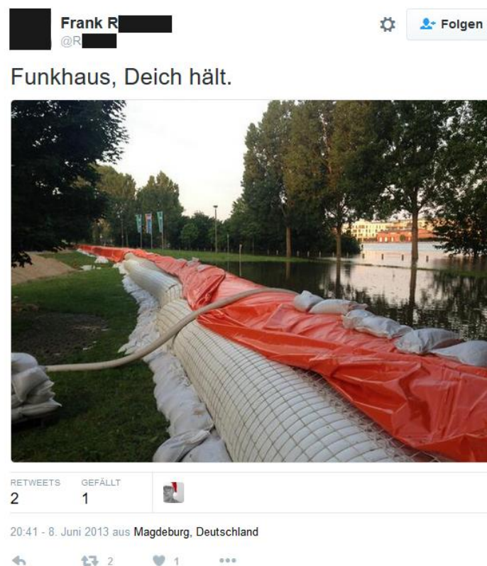
Figure 12. Tweet about the dike near the Funkhaus in Magdeburg 32
