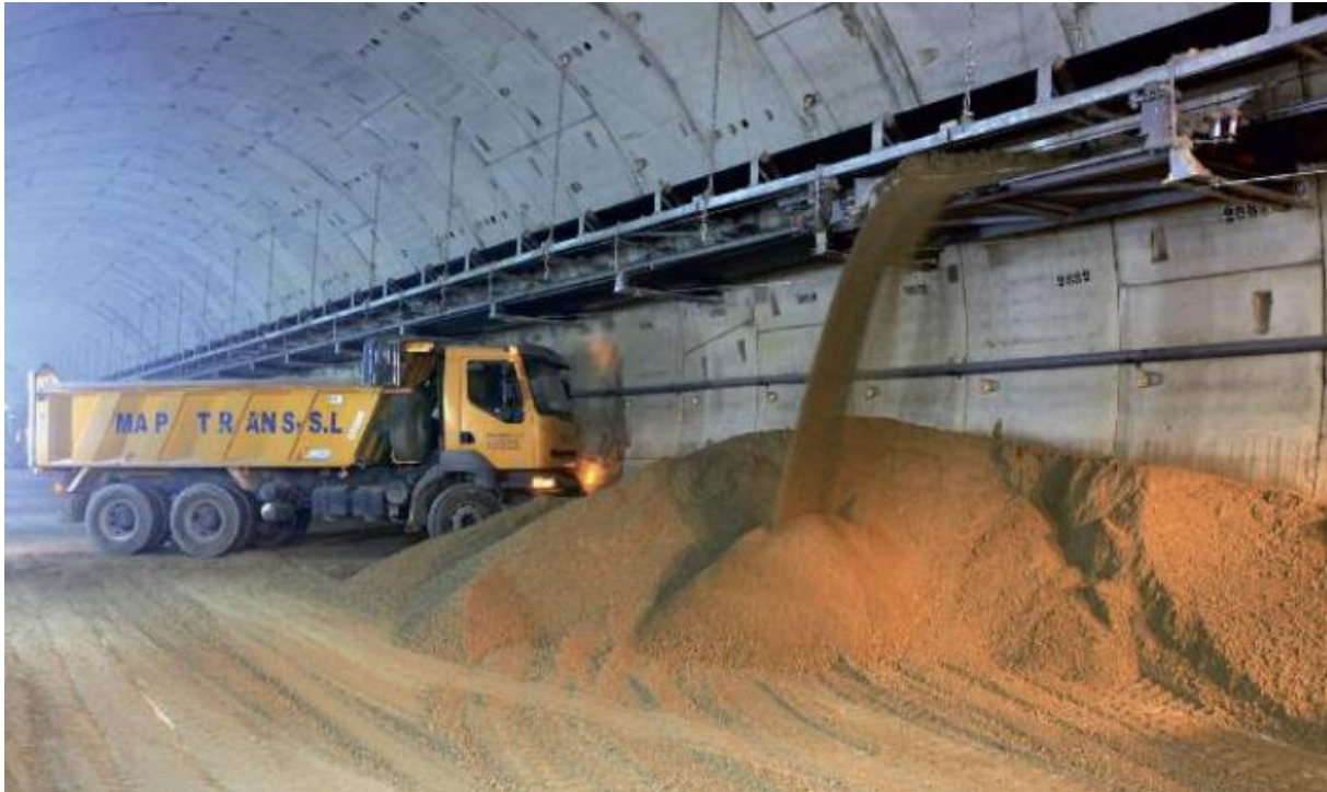
Figure 16: Muck removal using a conveyor belt system (Source: Own imagery)
