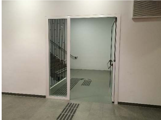
Figure 5.2.: Stairs in a distinct room on route 1
